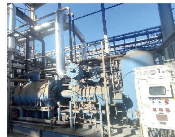
Low-temperature cascade unit of a polycrystalline silicon project
